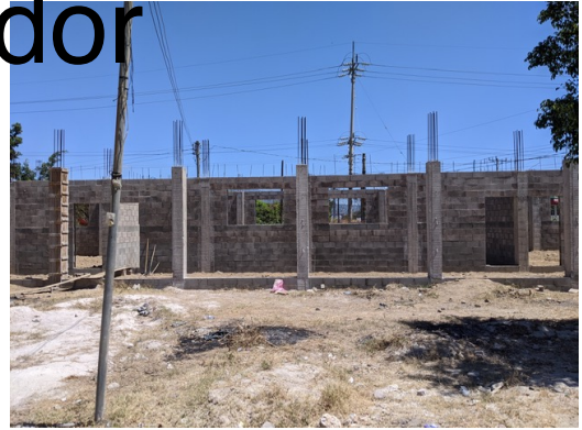
New school building under construction
